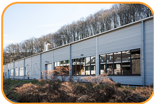
Rhodius Germany Plant
